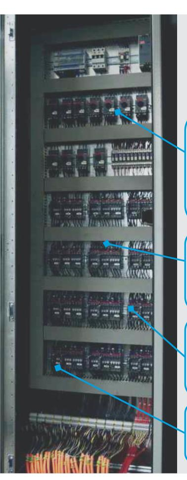
Automation panel is responsible for operating in accordance with the ventilation scenarios processed. PLC (Programmable Logic Card) which is carried by all mechanical devices (axial fans, jet fans, air / smoke dampers, doors etc.) in the system according to the signals coming from the carbon monoxide detection system and / or fire / smoke detection system which analyzes the situation in the parking lot.
